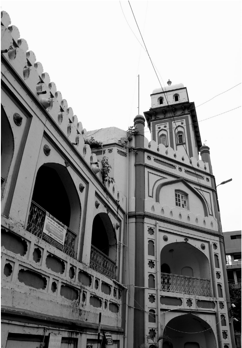
Figure 1.1 At the Gate of Mecca: Mughal hajj caravanserai, Surat, Gujarat, built in 1644. Built by the Mughal nobleman Ishaq Beg Yazid Haqiqat Khan (d. 1663–1664).
