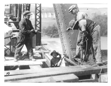
Figure 1. Rivetters building the Murray Bridge, New South Wales, early twentieth century. State Library of South Australia; image no SLSA: B 3161. Used with permission.
