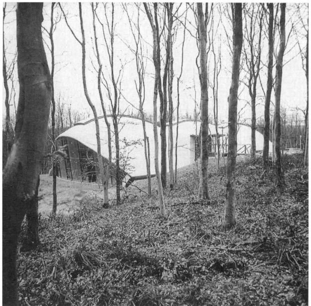
FIG. 2. The training centre built from spruce thinnings removed from Hooke Park during forest management.
