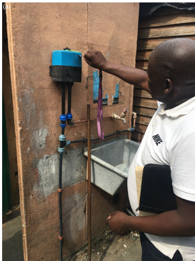
Figure 6a. Example of water meter installation within backyard area.
