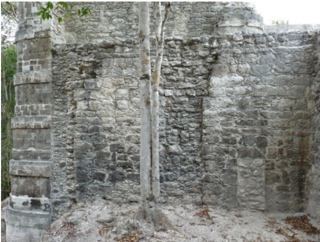
Figure 12. South (rear) side of the northwest tower of Structure 5N2 where unfaced parts of wall are visible. These were surely intended to receive perpendicular walls, which were never actually built. Photo courtesy of the Río Bec Project.
