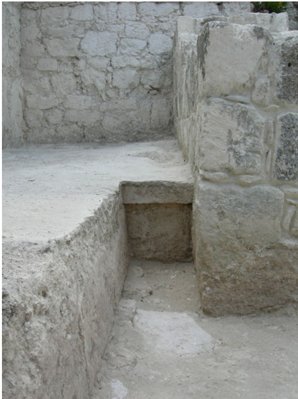
Figure 6. Raised "floor" of Room c without stuccoed surface. Note also the absence of a salient band at the edge of the upper level, except on the small sides. Photo courtesy of the Río Bec Project.
