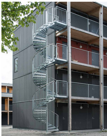
Figure 1. Photo of a manufactured spiral staircase, consisting of 3 segments. Reproduced from Weland AB (2016) with permission.
