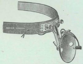
An improved lamp on the Klar principle; fitted with unbreakable mirror of speculum metal; easily adjusted and economical in use. (Vide Lancet, March 13th, 1920.)
