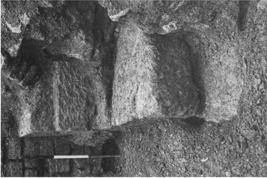
B CIRENCESTER Bastion 4, south side (p. 237). CULLEN, CIRENCESTER: RESTORATION OF TOWN WALL.
