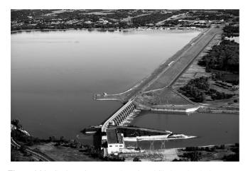
**Figure 4.21.** Gavins Point Dam and Lewis and Clarke Lake, the lowermost dam on the Missouri River. The structure is an embankment dam of earthen and chalk-fill materials. Dimensions: closure in 1955, upstream drainage: 723,825 km<sup>2</sup>, 23 m high, 2,650 m long, total reservoir capacity is 606,873 m<sup>3</sup>, surface area of 12,700 ha, depth of 14 m, and maximum length of 40 km. (Photo and data source: U.S. Army Corps of Engineers.)
