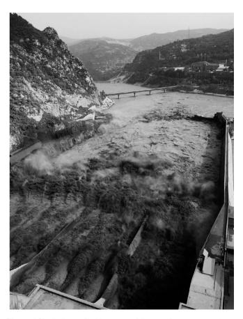
**Figure 4.52.** Sediment flushing event of Sanmenxia Dam, Huanghe River. Sanmenxia Dam closed in 1960 and is the first main-stem dam on the Huanghe River (contributing drainage area 688,400 km<sup>2</sup>). (Photo date: July 26, 2013. Source: R. Mueller, licensed by CC.)
