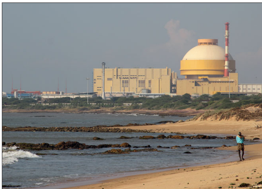
The Kudankulam Nuclear Power Plant
