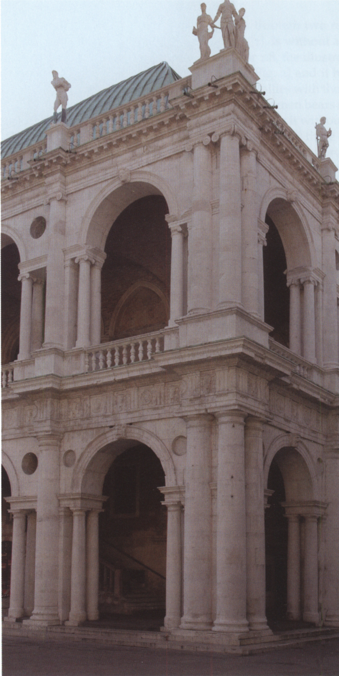
Fig. 7. Palladio's Doric and Ionic orders: arcades (northwest corner) of the Basilica, Vicenza
