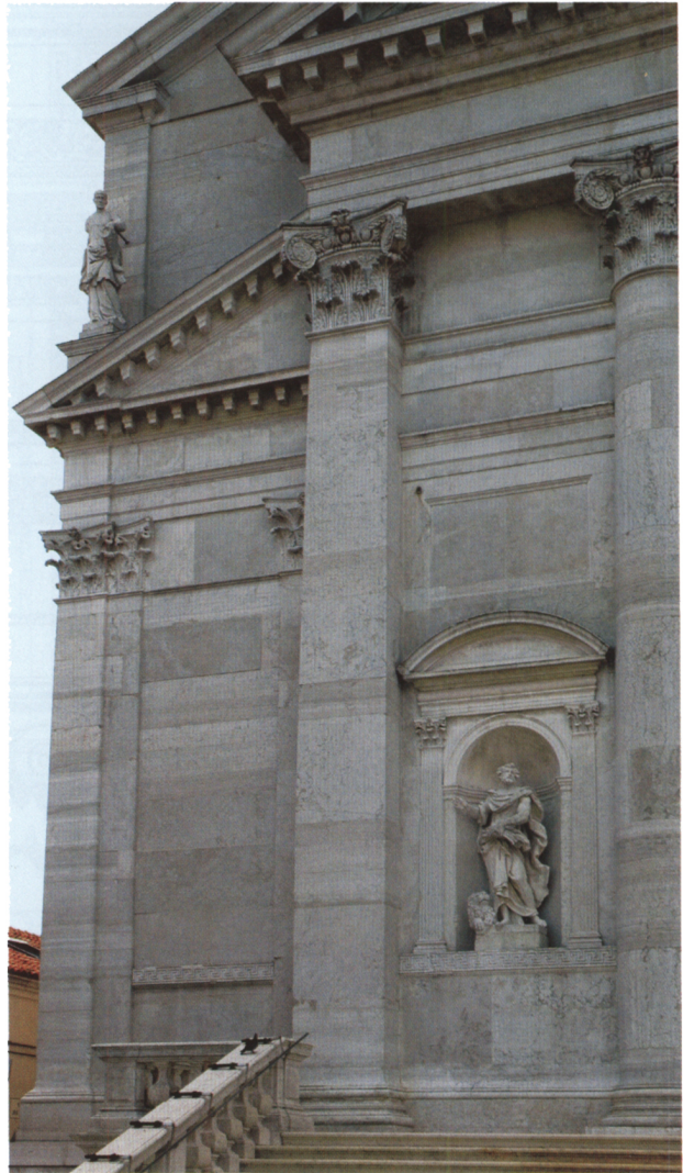
Fig. 16. Palladio's Corinthian and Composite orders: façade of the Redentore, Venice
