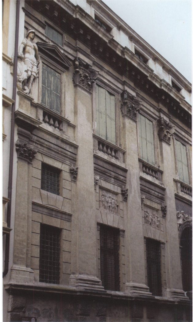
Fig. 18. Palladio's Corinthian and Composite orders: façade of Palazzo Valmarana, Vicenza
