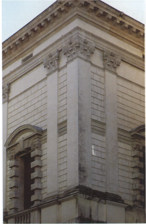
Fig. 20. Palladio's Ionic and Composite orders: exterior (northeast corner) of Palazzo Thiene, Vicenza
