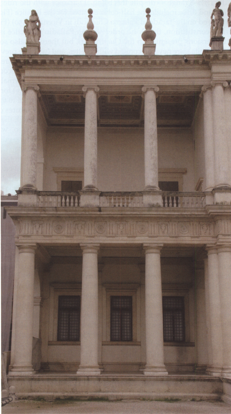
Fig. 8. Palladio's Doric and Ionic orders: façade (first-executed southern portion) of Palazzo Chiericati, Vicenza
