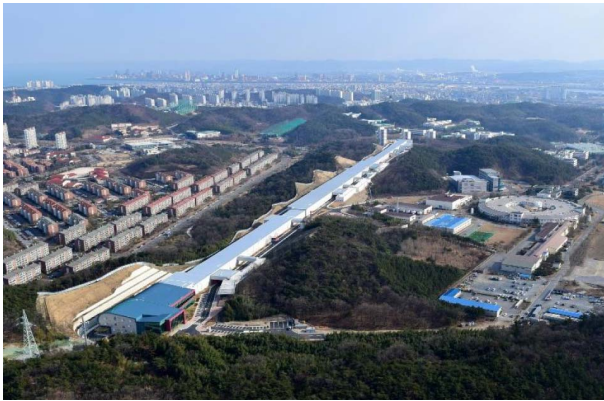
Figure 1. Construction site of PAL-XFEL.
