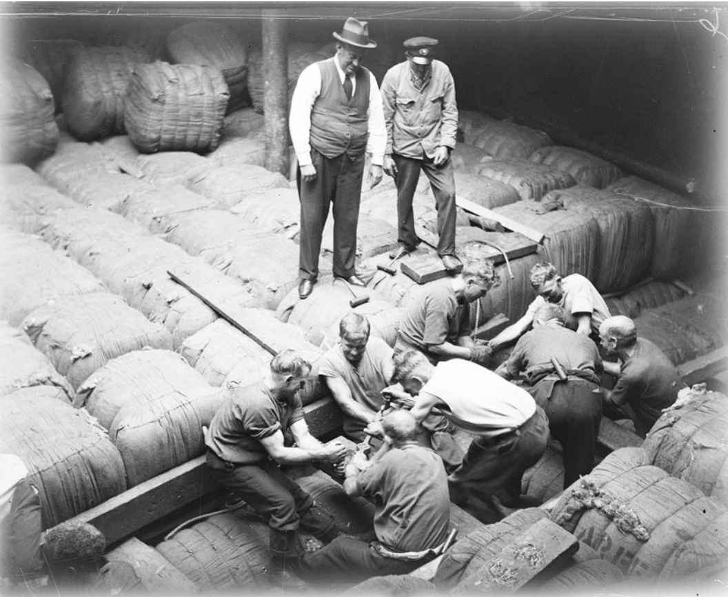
Figure 4. Wool screwing in the barque Magdalene Vinnen , Sydney, 1933. Australian National Maritime Museum Collection. 00035587. https://www.flickr.com/photos/anmm_thecommons/7104626313 . Public domain.
