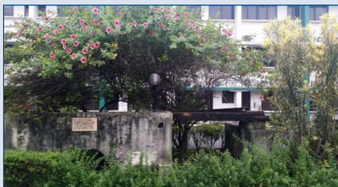
Entrance to the Yaba Hospital, Lagos, with remnants of the first hospital building on this site.
