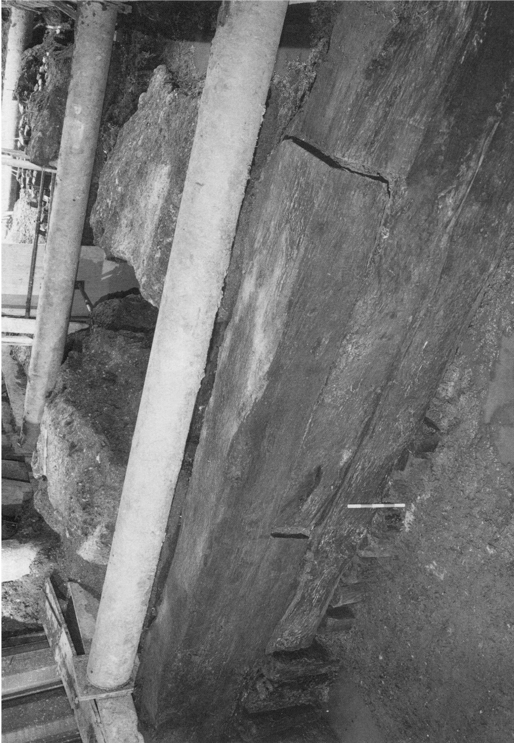
London, Canon Street Station: timber revetment of the east bank of the mouth of the Walbrook (p. 270). (Photo: Museum of London)
