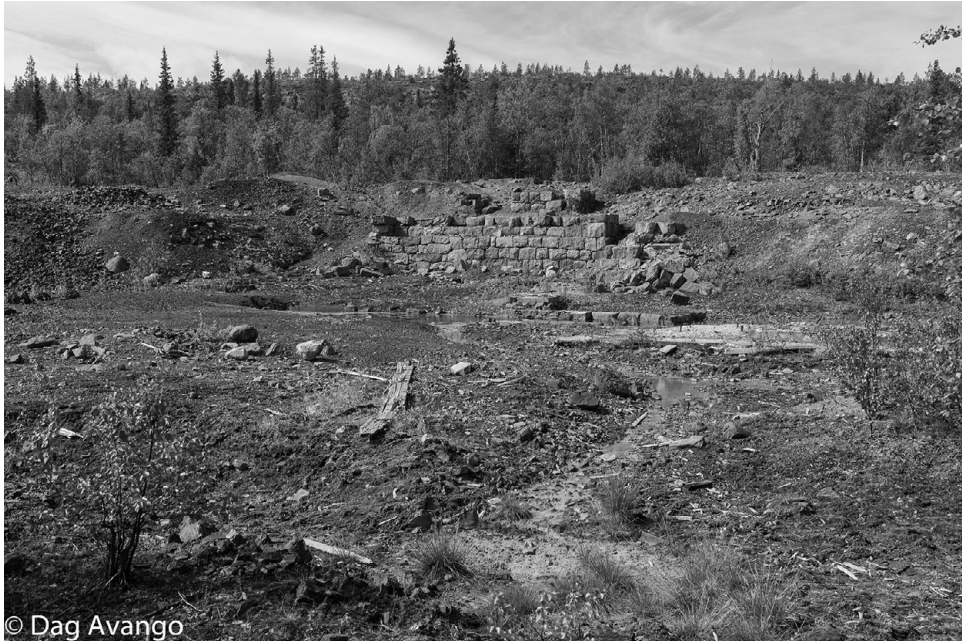
Figure 9.6 The contaminated remains of the Nautanen concentration plant and copper smelter. Photo by Dag Avango
