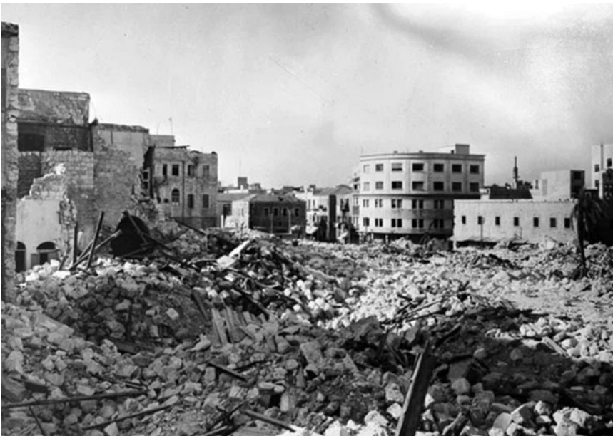
FIG. 1 View of the destruction of the Old Town. Photograph by Jim Pringel, public domain.
