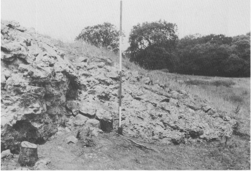
A. Lympne. Bastion 9: looking north. The facing-stones survive to the left of the rod (p. 233).
