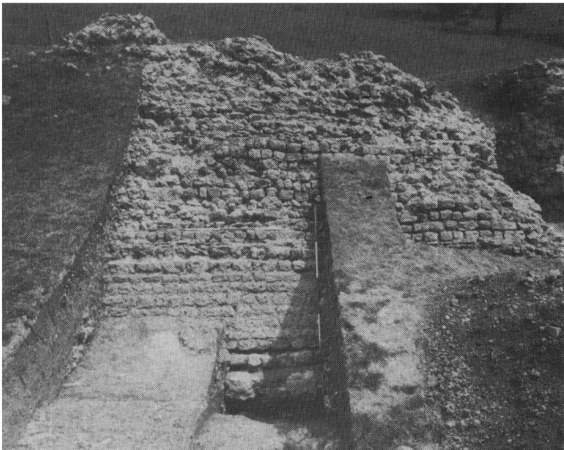
B. Lympne. The east wall in trenches 4 and 6. Facing east (p. 251).
