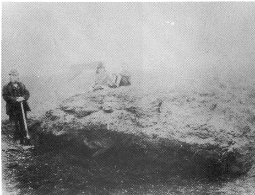
A. Destruction of Fen Causeway in the peat Fen between Whittlesey and March, c. 1905. Note a fragment of the timber corduroy beneath the road make-up (p. 131).
