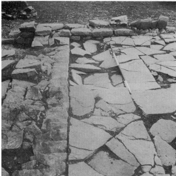
B. Bradley Hill: Building 1, Room 2, showing original SE corner, looking S. (p. 183).
