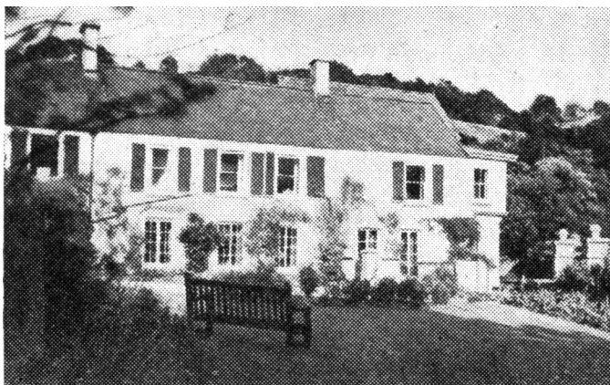
CRICKLEY COURT—ONE OF THE SEPARATE VILLAS
