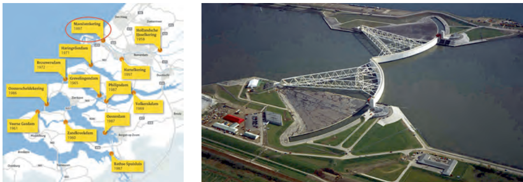
Figure 1.5 Left: The original 13 storm dikes and barriers from the Delta Works. Right: The Maeslantkering when closed. Sources: © Rijkswaterstaat (left) and Watersnoodmuseum (right)
