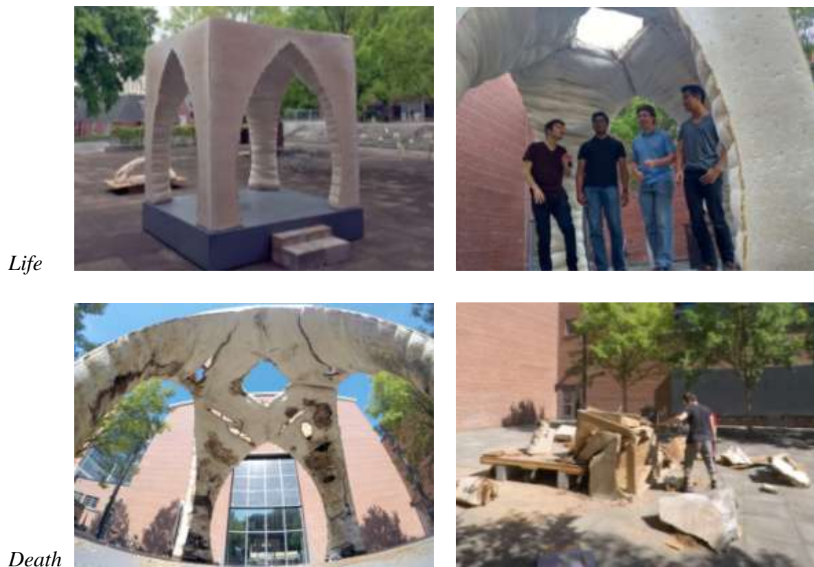
Figure 1. Life and death of Monolito Micelio: a monolithic pavilion for a singing performance. The structure was cultivated from a single colony of mycelium in a hemp substrate. After the performance, the structure was left to decay and eventually broken down, disposed, and “fed” to compost. Photos by Jonathan Dessi-Olive.
