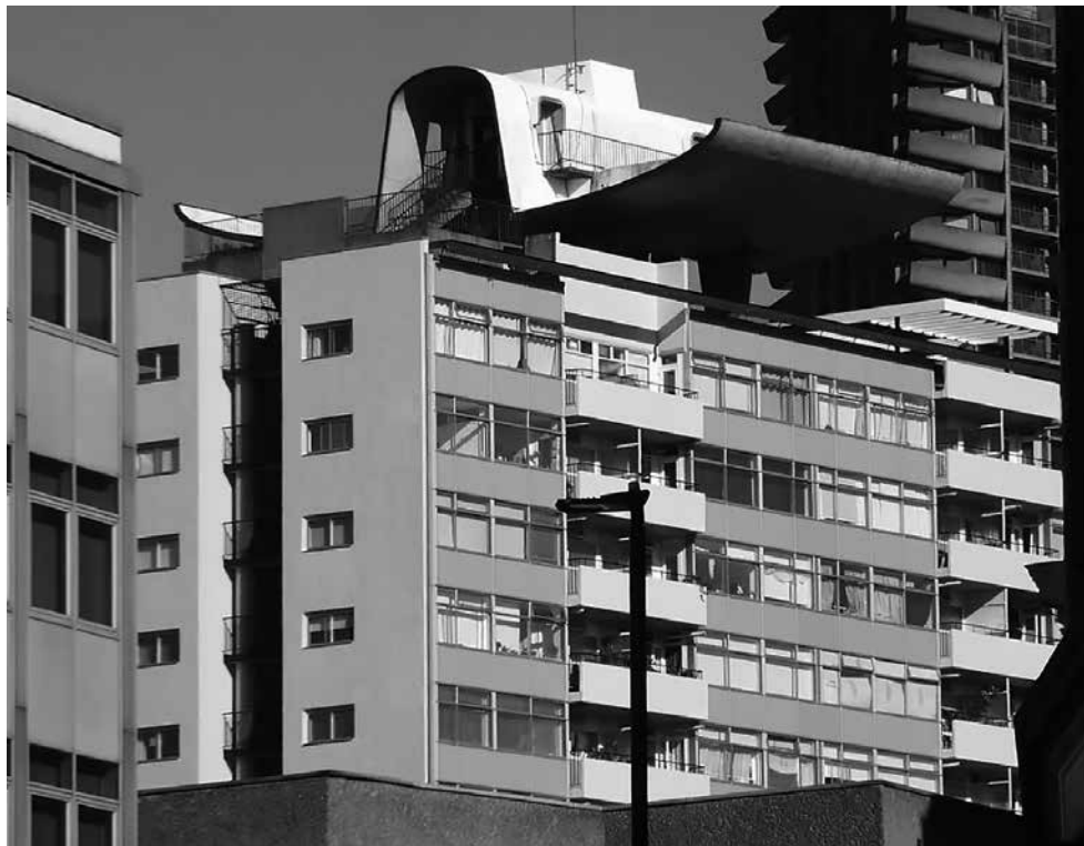
4 Roof detail of Great Arthur House, Golden Lane Estate, Chamberlin, Powell and Bon, completed 1957.
