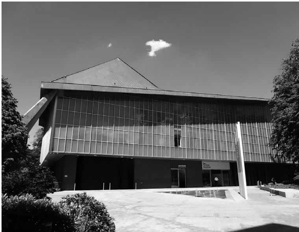
7 Commonwealth Institute, now Design Museum, Kensington High St, RMJM, completed 1962.
