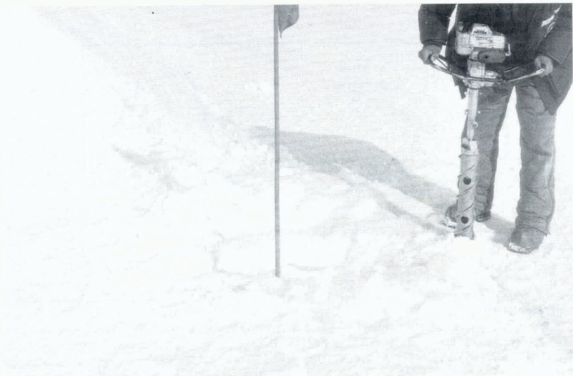
Fig. 3. Site of an ice failure caused during proof-rolling.
