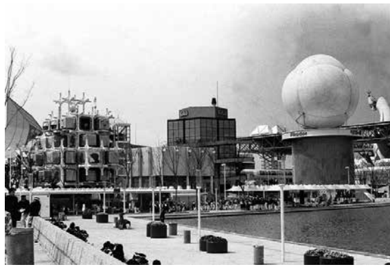
2 Osaka Expo '70. Right (background): Kenzo Tange's Big Roof. Left (foreground): Kisho Kurokawa's Takara Beautilion. Both structures demonstrate the Metabolist commitment to adaptable, modular structures into which pods could be inserted to serve various uses.
