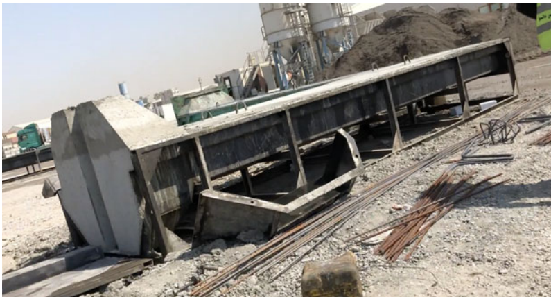
Figure 2. A t-wall in its mold, northern Iraq, 2021. Photograph by the author.
