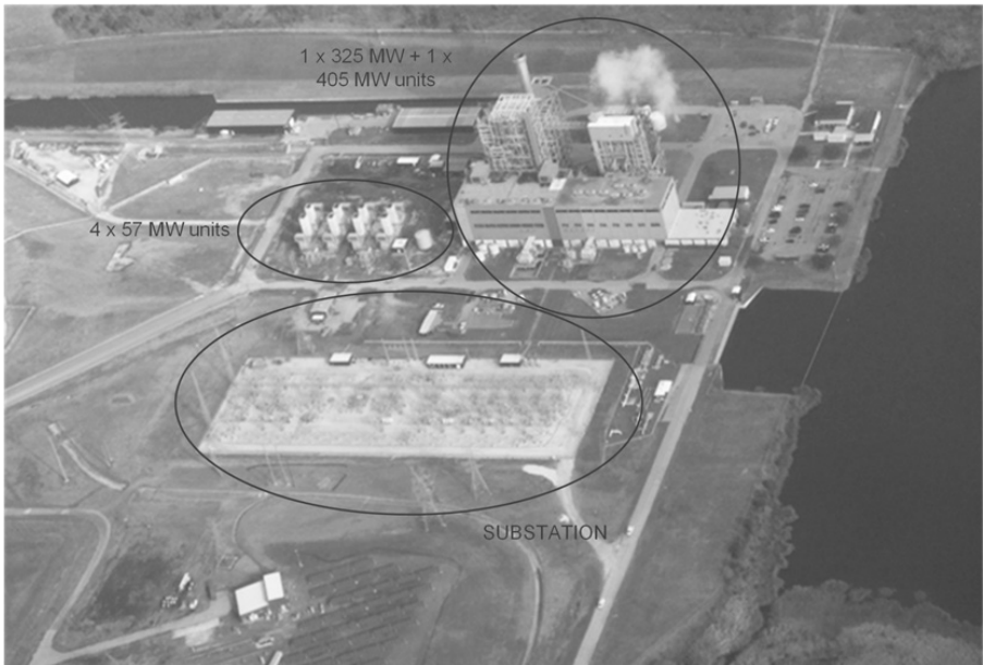
Figure 2.10 The Decker Creek power station with a total capacity in its natural gas turbines of 958 MW. The photovoltaic system at the bottom of the image has a capacity of 300 kW and has about the same footprint as the four 57 MW natural gas turbines.
