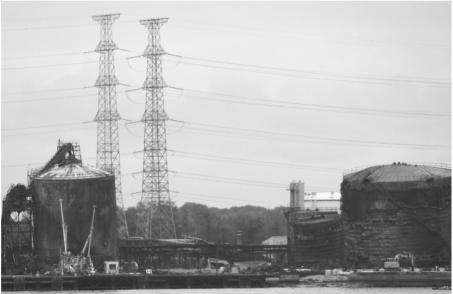
Figure 2.25 Anchor lattice towers in the port of Sendai, Japan. The tanks in the foreground were damaged during the tsunami of March 2011.
