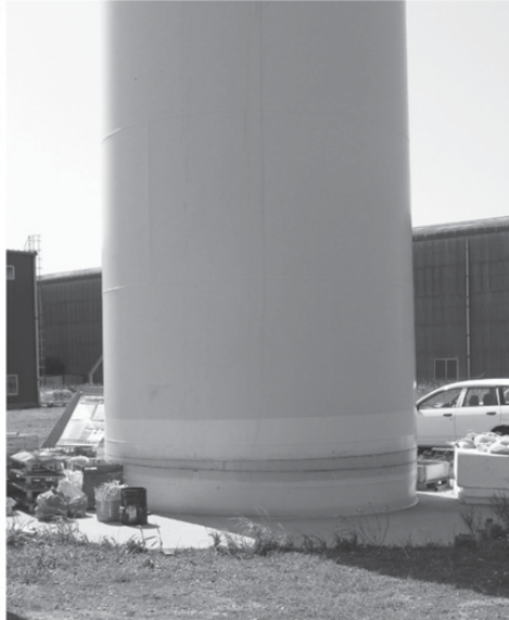
Figure 2.95 A wind turbine that tilted during the 2011 earthquake in Japan. A ring was added at the base to compensate for such tilt (see (b)).
