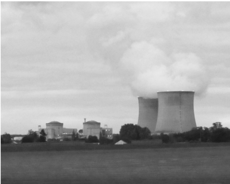
Figure 2.18 The Saint Laurent Nuclear Power Plant. The buildings for its two reactors, each producing 956 MW of electric power, are seen to the left of the image center.
