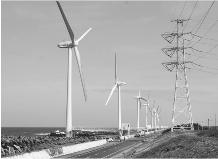
Figure 2.94 Wind turbines undamaged by tsunami waves in Japan after the 2011 earthquake.
