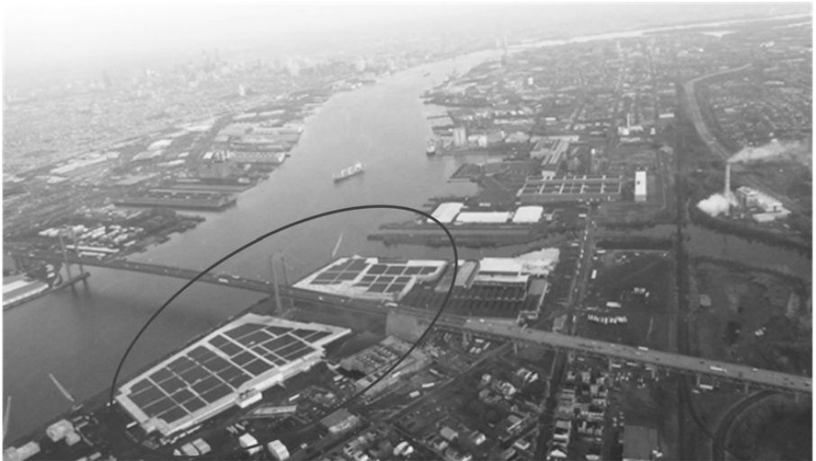
Figure 2.5 The Gloucester Marine Terminal photovoltaic power plant.
