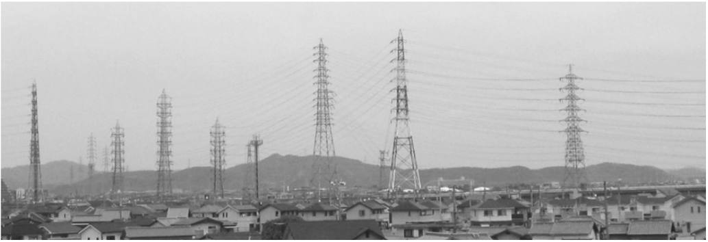
Figure 2.22 Overhead high-voltage transmission lines in a dense urban area.
