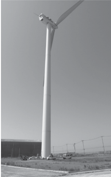
Figure 2.95 A wind turbine that tilted during the 2011 earthquake in Japan. A ring was added at the base to compensate for such tilt (see (b)).
