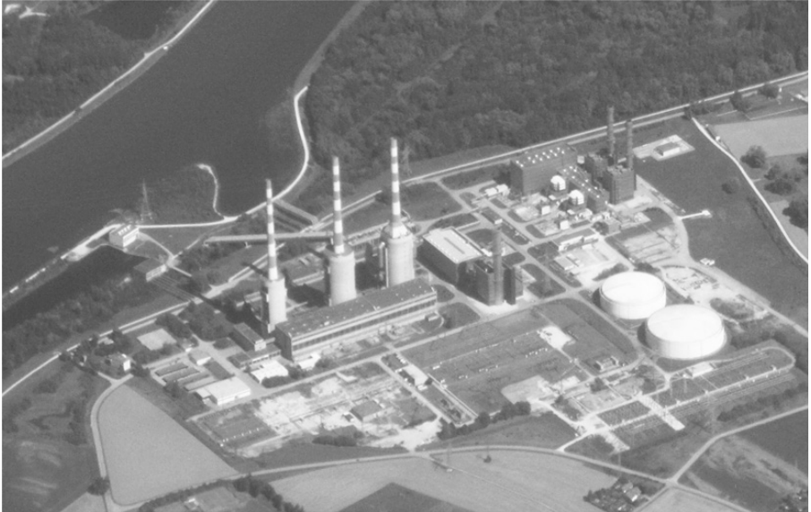
Figure 2.12 Irsching Power Station, which operates five power generation units: Unit #1 of 150 MW, Unit #2 of 330 MW, Unit #3 of 440 MW, Unit #4 (in one of the darker buildings at the center of the image to the right of the three stacks for units #1 to #3) of 569 MW, and Unit #5 (on the top right in the other, darker building) of 860 MW. Both units #4 and #5 operate in a combined cycle.
