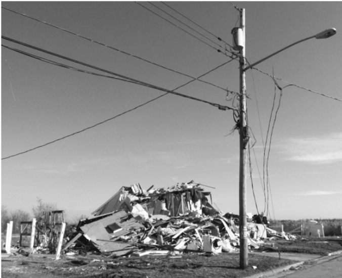
Figure 2.90 Storm surge damage to buildings may be different from effects on built infrastructure components.
