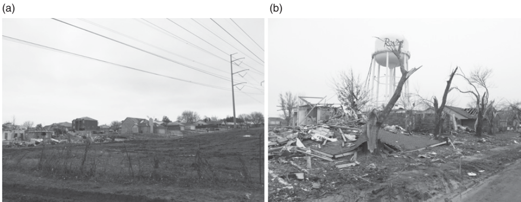
Figure 2.98 Example of damage caused by a tornado. (a) Destroyed dwellings next to a seemingly undamaged transmission line. (b) An area completely destroyed by a tornado.
