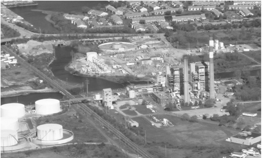
Figure 2.11 E. F. Barrett Power Plant, which is comprised of two 195 MW dual-fuel steam units and eleven simple-cycle, dual-fuel combustion turbines, which are divided between fifteen 15 MW and four 40 MW combustion turbines.
