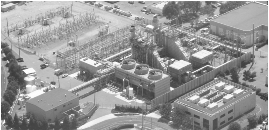
Figure 2.7 The Donald Von Raesfeld Power Plant equipped with two 50 MW natural gas-fueled combustion turbines and one 22 MW steam turbine.
