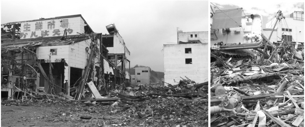
Figure 2.91 Damage caused on poles by debris carried by tsunami waves.
