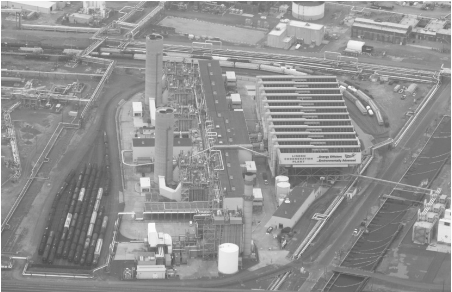
Figure 2.8 The Linden Cogeneration Power Plant.
