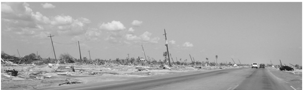
Figure 2.89 Example of intense storm surge damage.
