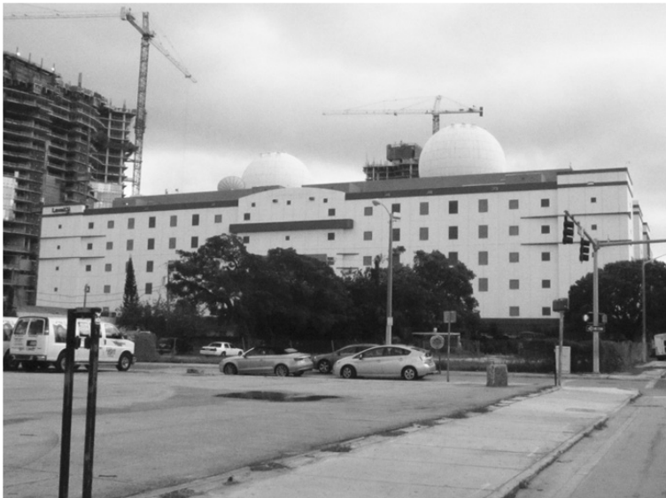
Figure 2.53 The building of the NAP (network access point) of the Americas.
