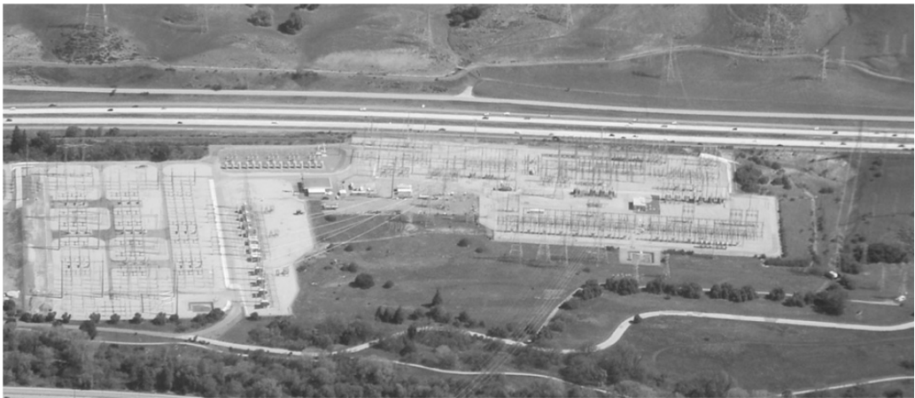
Figure 2.35 Aerial view of the Metcalf substation in California.
