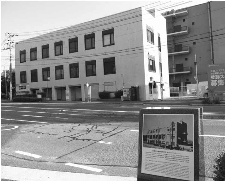
Figure 2.101 NTT West telephone central office in the city of Hiroshima as seen today and two months after the nuclear explosion in 1945 on the plaque at the bottom right of this image. Although this central office was one of the very few surviving buildings within a one-mile radius from the explosion, it still sustained damage to its equipment.
