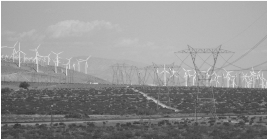
Figure 2.6 Part of the San Geronio Pass wind farm (installed capacity of 615 MW) with one of the transmission lines used to connect it to the load centers.
