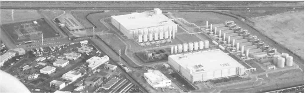
Figure 2.52 Google's data center in Henderson, Nevada. The main electric substation is seen on the top left and a secondary substation is observed between the two buildings. Cooling and power backup equipment is seen between the two buildings and on the right.
