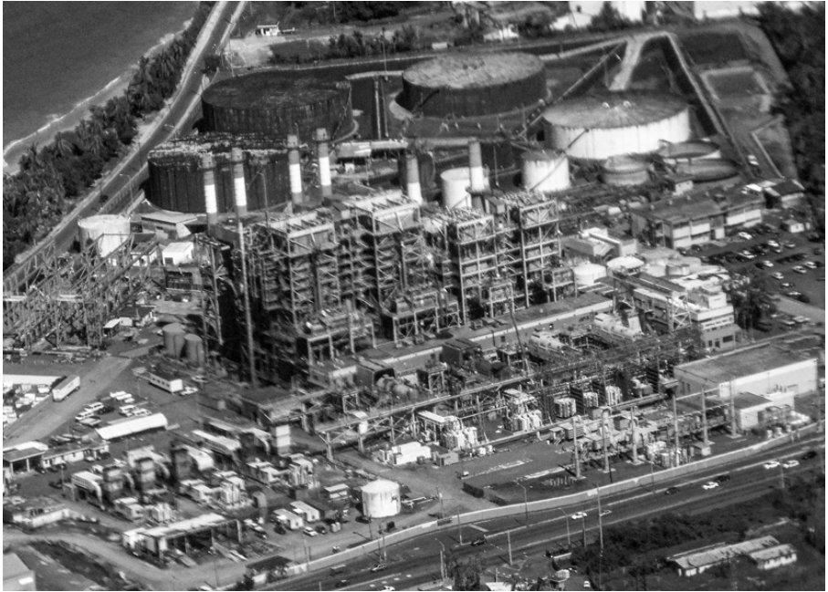
Figure 2.13 Palo Seco Power Station, which uses Residual #6 (fuel oil) that is stored in the tanks shown in the upper portion of this image. This power station is equipped with two 85 MW and two 216 MW turbines for a total capacity of 602 MW.
