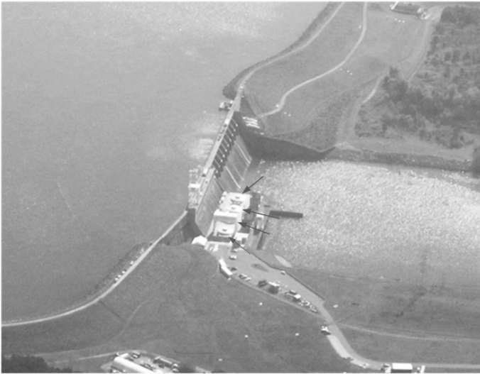
Figure 2.2 Cowans Ford Hydroelectric Station. The arrows indicate the location of its four turbines.
