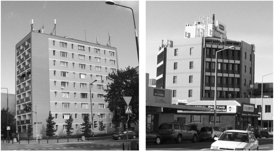
Figure 2.78 Two examples of rooftop-mounted cellular antennas.
