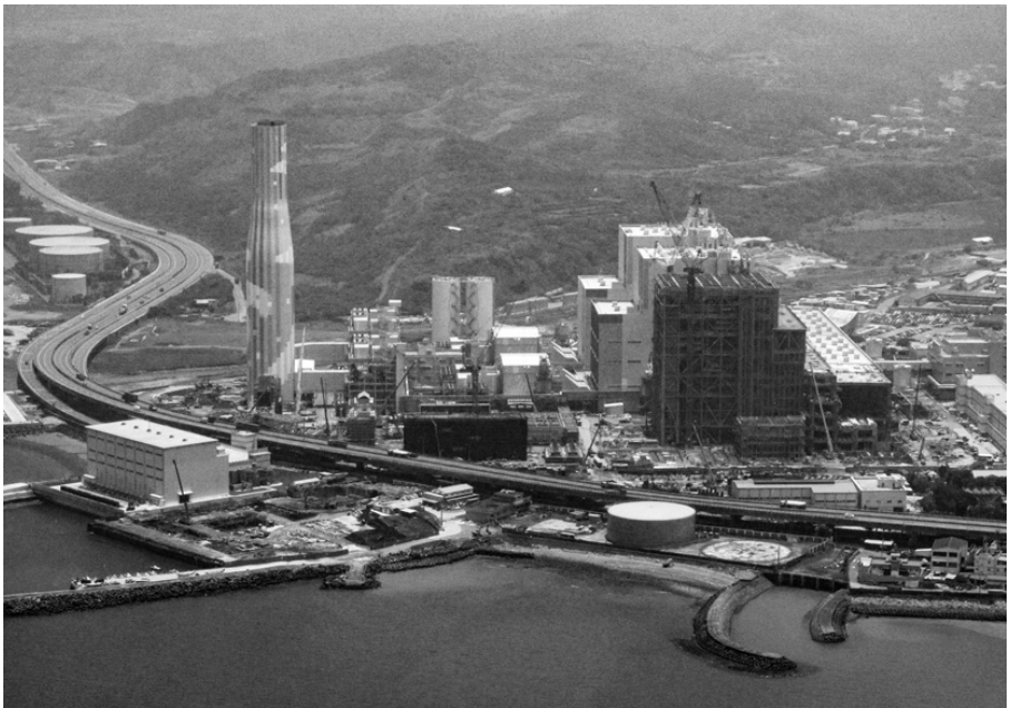
Figure 2.15 The Linkou Power Plant in Taiwan operating with two 800 MW coal-fired units while a third 800 MW unit was being constructed.
