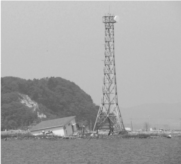
Figure 2.96 A destroyed building partially sunk due to ground scour caused by tsunami waves.
