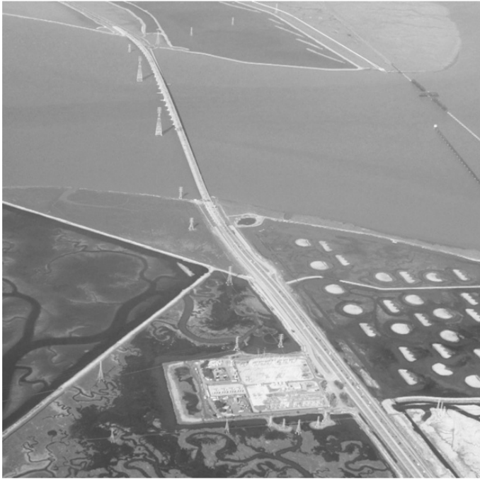
Figure 2.26 A transmission line end at a substation is seen at the bottom of this image.
