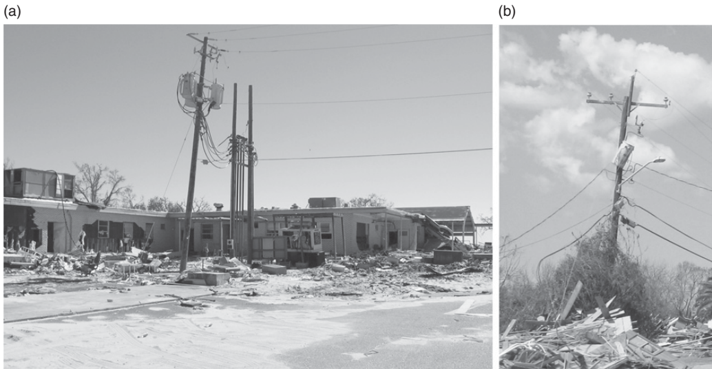
Figure 2.45 Pole-mounted transformers after suffering a storm surge. (a) Surviving transformers. (b) A damaged transformer but still mounted on the pole.
