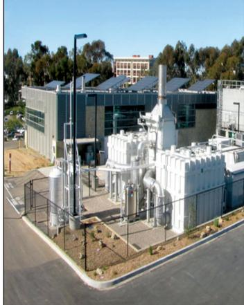
Fuel-cell-based power systems can be designed for high efficiency that can be further improved by hybridization. Efficiency improvements in solid-oxide fuel-cell/gas turbine hybrid systems are estimated to be exceptionally high. These hybrids can be incorporated into coal-based power plants to form a power system referred to as an integrated gasification fuel-cell system.
