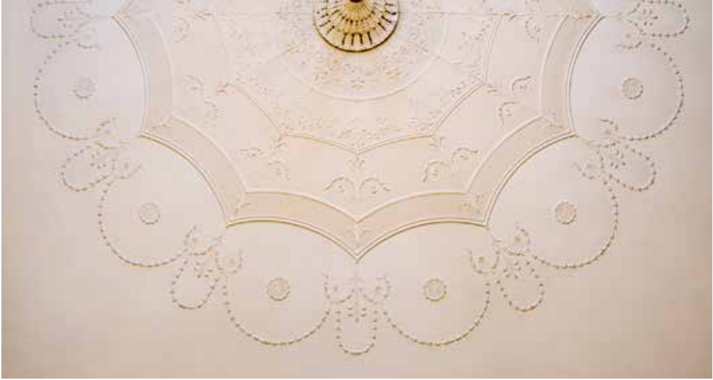
Fig. 8. Ceiling of front first-floor room (detail) at 17 St Stephen's Green, Dublin, created by Michael Stapleton, c. 1778, photograph by Stephen Farrell of 2007
