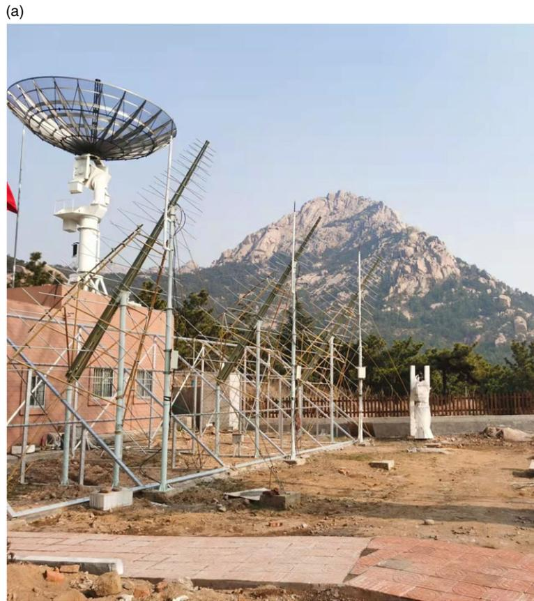
Prototype of the antenna array receiving system.
