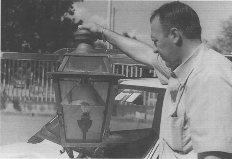
Figure 2. Modification of an open lantern “old style” with a cheap and functional conical metal screen. Dispersion flux is reduced by 50%. Cost: US$5 each.
