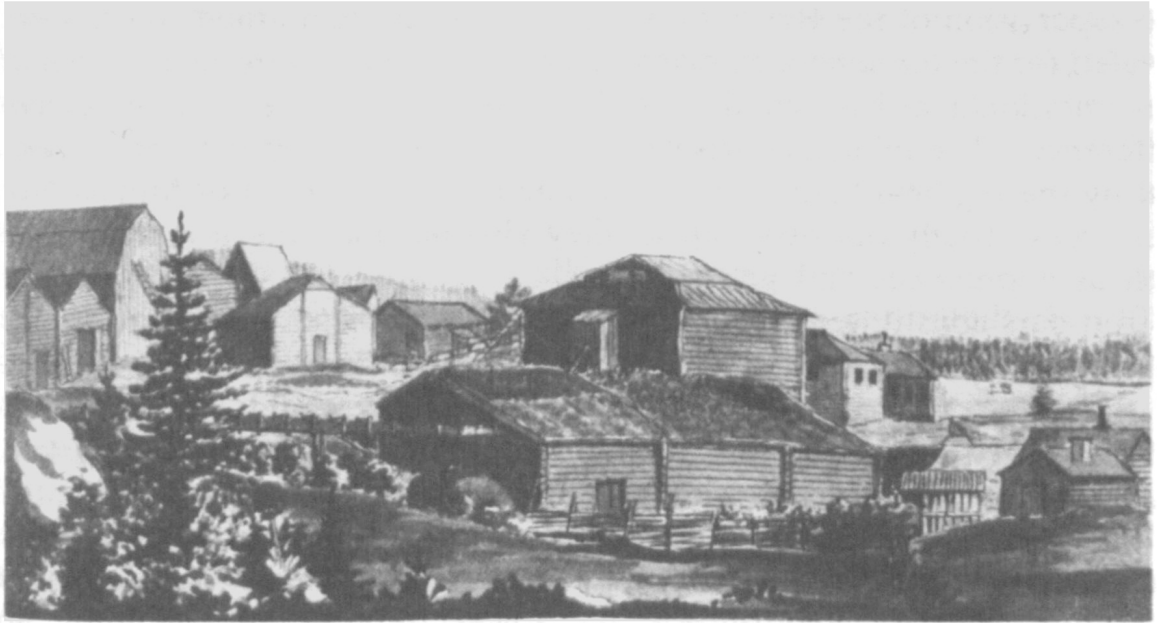
Figure 2. The Greksåsar village in the mining district of Nora (Bergslagen) in 1846. The blast furnace is situated in the centre and the smaller buildings surrounding it are stores for iron and charcoal. The drawing gives an impression of the spatially dispersed and socially differentiated Swedish industry in contrast to the centralized uralian premises. (Photo: Jernkontoret's bruksbildskatalog)
