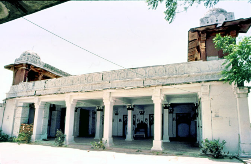
Figure 11. (Colour online) Mosque of Bībī Zarrīna, view from the courtyard looking west. The crenulations reflect the pattern of those of the tomb, but those above the front façade are carved on panels and those of the upper colonnades are each carved on a separate slab. The game of similarity and contrast between the tomb and the mosque is maintained in every detail.
