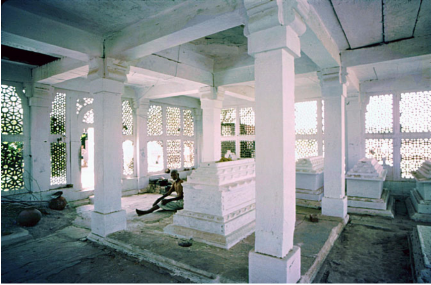
Figure 6. (Colour online) Tomb of Bībī Zarrīna, interior. View looking north-west showing the fine pierced stonework (now whitewashed) surrounding the cenotaph, and the raised roof over the Bībī's tomb.
