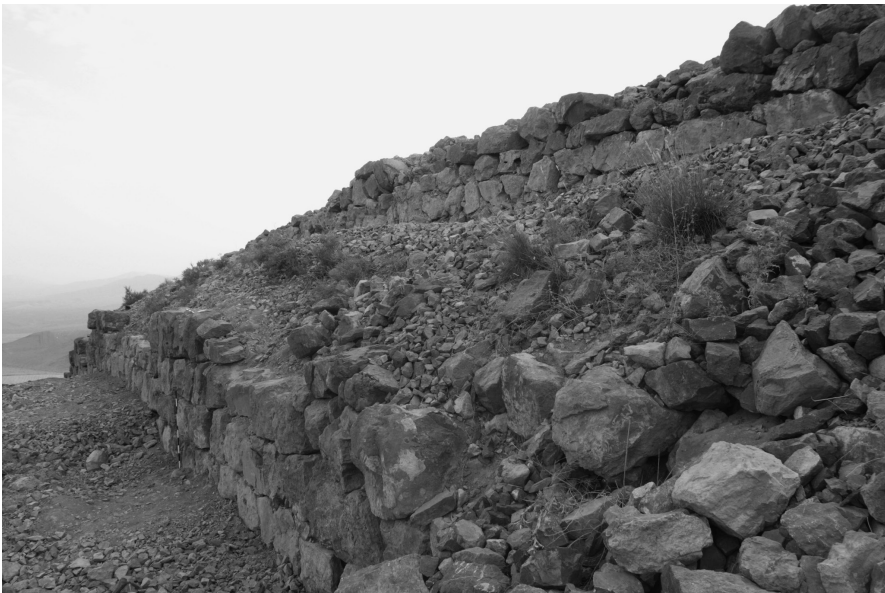
7.6. Western wall of the northern administrative building. Photograph by the Naxçıvan Archaeological Project.
