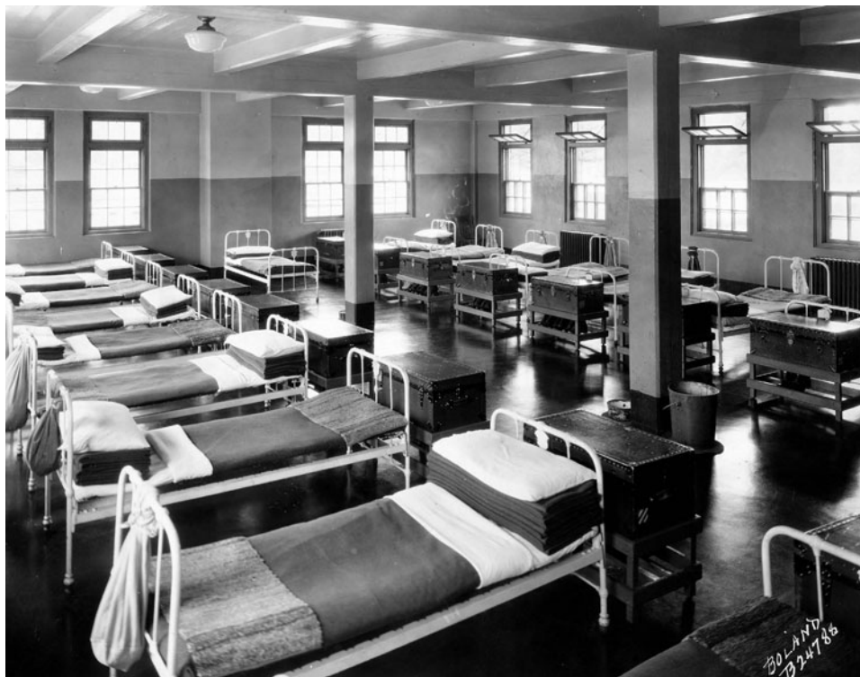
Figure 1. A typical open-bay barracks configuration circa 1935. Source: Joint Base Lewis–McChord (JBLM) Historical Archives, cataloged by Historical Research Associates.
