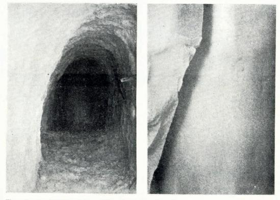
Fig. 4. Present end of Silbersatted tunnel (61 m. long in 1952.) Fig. 5. Open crack in tunnel 61 m. below surface (See text pp. 195 and 196) Photographs by J. E. Fisher
