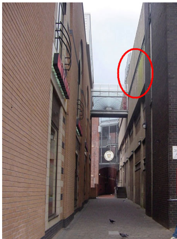
Fig. 2. Contemporary photograph of alleyway outside Forum 28 into which droplets of contaminated water were emitted. Red circle indicates the vent from which the Legionella -contaminated aerosol came. (Copyright © Dr Nigel Calvert, NHS Dumfries & Galloway.)
