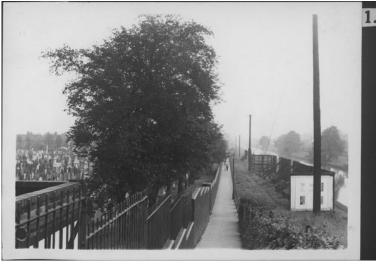
Figure 7—Bridgwater Canal, view from hill, TNA ASSI 84/242.
