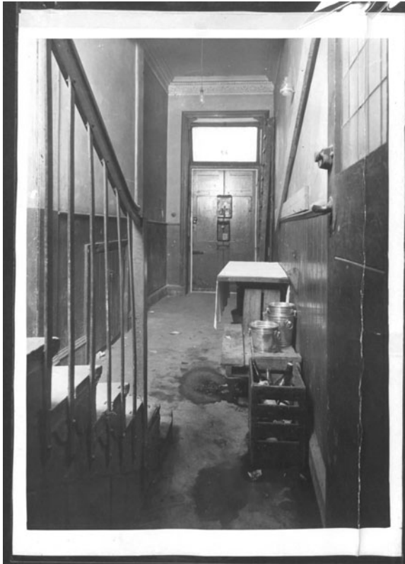
Figure 3—Rear of Bellometti's Restaurant, Soho, view from staircase, TNA CN 27/10.
