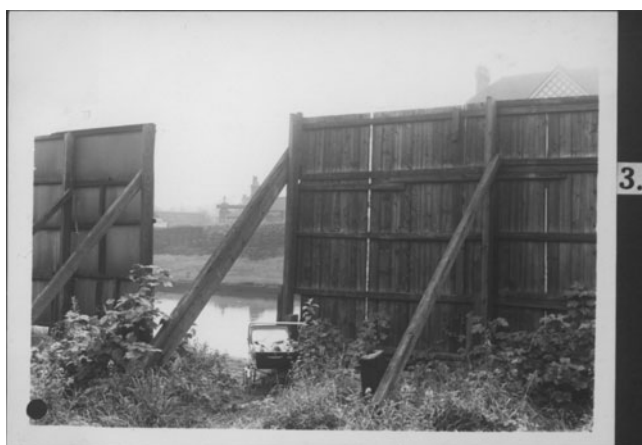
Figure 8—Bridgewater Canal, view from path, TNA ASSI 84/242.
