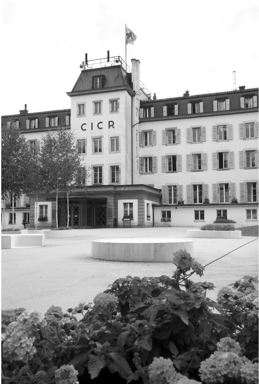
Photograph 1.1 ICRC headquarters, Geneva, main building, as of 2013. Formerly the Carlton Hotel built in 1876, the building with its majestic views was made available to the ICRC by the city of Geneva in 1946. Between 1863 and 1946 the ICRC operated out of different premises in Geneva.
