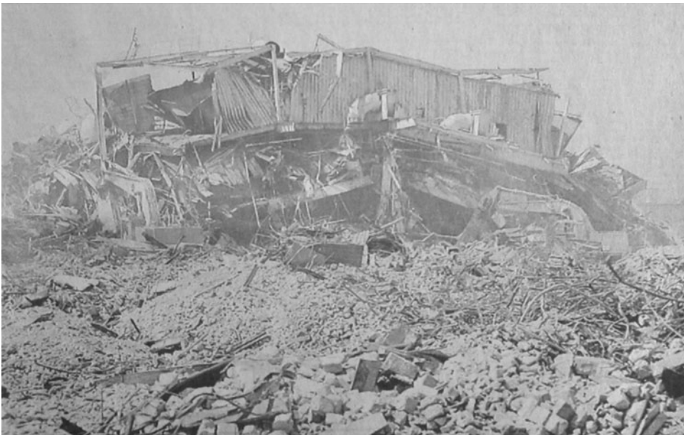
Figure 7. Photo of the demolished auto plant from the Valley Daily News . “Van Nuys Plant 8000 Van Nuys Blvd 91409” Facebook Group.
