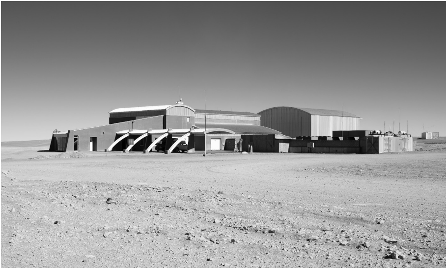
Figure 9.5 The AOS Technical Building. The arches in the foreground are vehicle shelters. The large shed in the background to the right is the transporter shelter. Credit: ESO, CC BY 4.0.
