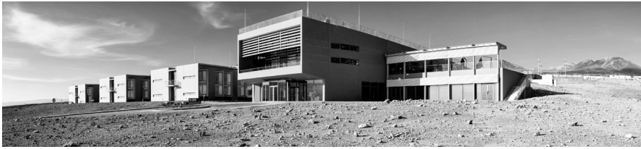
Figure 9.6 The ALMA residence hall provides living accommodations for up to 120 staff members and visitors along with a cafeteria, and a variety of venues for exercise and relaxation. Credit: ESO, CC BY 4.0.
