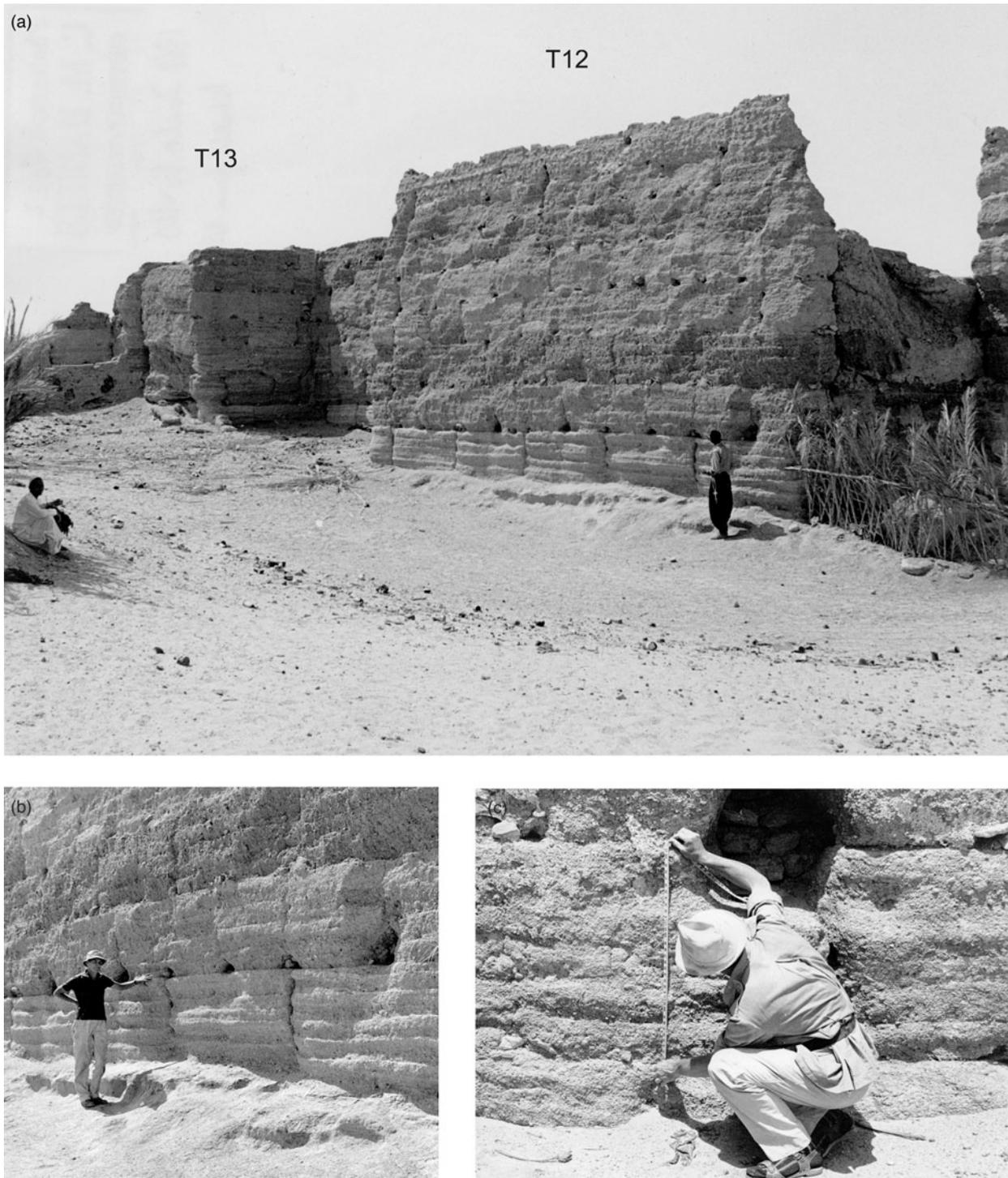
Figure 7. Details of pisé construction: a) north wall, near north-west corner tower 12, showing courses of pisé blocks (note different colour of foundation layers); b) close-up of pisé blocks showing putlog holes with stone lining; c) close-up of internal layering of rammed earth construction for each block.
