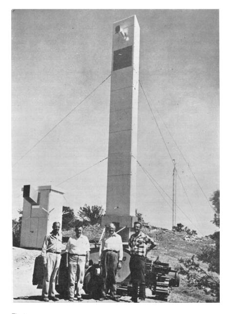
Fig. 42. — Photograph of the seeing test towers located on Kitt Peak. Polaris monitor telescopes are located in both the 10-foot and 60-foot towers. Microthermal probes project out the north face of 60-foot tower near the top and bottom. Note the outriggers supporting the outer tower shell. Shown are Drs. E. F. Carpenter, F. K. Edmondson, J. C. Duncan and A. B. Meinel.
