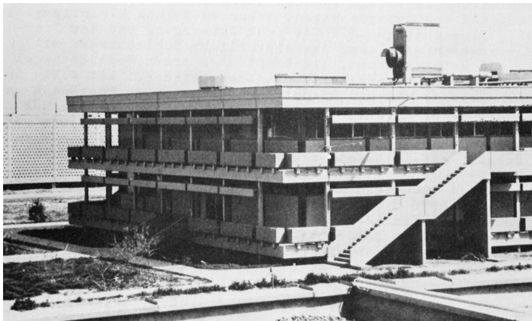
Figure 4. The canteen building after completion at the Baghdad slaughterhouse compound. Ipro-Dessau (German Democratic Republic). 'VEB Industrieprojektierung Dessau: Betriebschronik', vol. 2, n.d.
