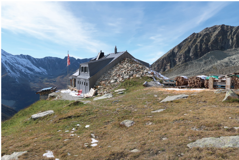
Figure 3. Photograph of a snow avalanche defence built against the Cabane Arpitettaz near Zinal, Switzerland. The geometry of boulders built up against the structure resembles a maximal pile (§ 7), which is a stable shape that effectively diverts incoming snow away from the building.
