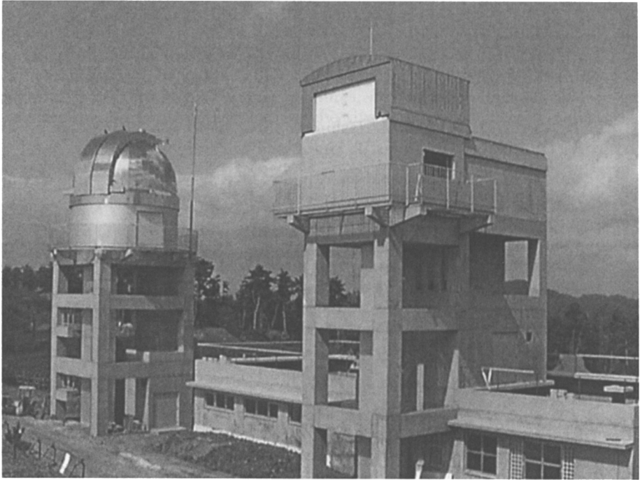
Figure 1. An over-view of the Bisei Spaceguard Center. A 1-m telescope will be set in the dome and the 25-cm and 50-cm telescopes are operated in the sliding roof building.
