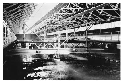
Figure 1b Model ship in towing tank
