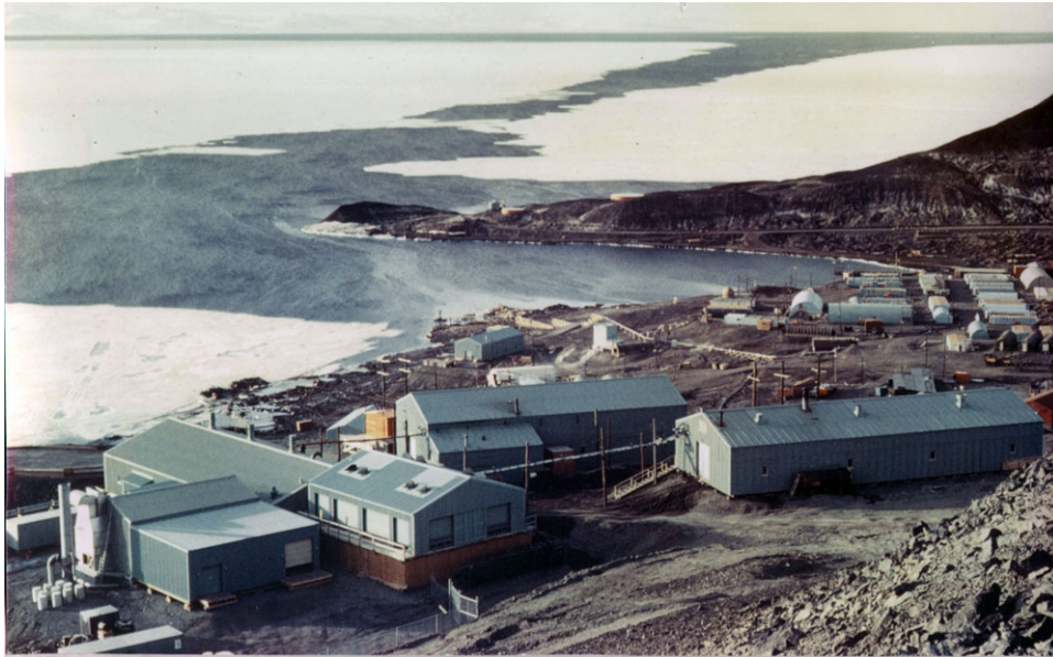
Figure 2. Photo of PM-3A Nuclear Power Plant, 1965. United States Antarctic Program, Antarctic Photo Library, Photo taken by US Army Engineer Research and Development Labs, NSF. Public Domain.
