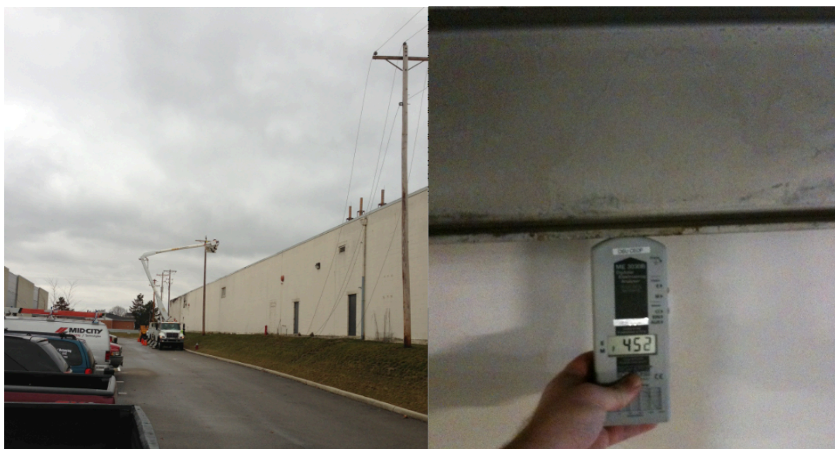
Figure 2. Relocation of power lines adjacent to new CEMAS, performed by local utility (Left). Magnetic fields from power lines inducing current in building steel as evidenced by field survey work (Right).
