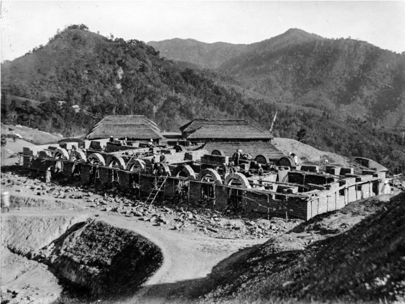
Figure 1.17 The Quarter Guard under construction in Aijal, 1896. SA.
