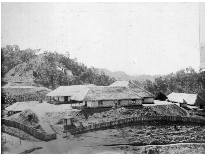
Figure 1.16 A bungalow section of Fort Aijal, c. 1892. KPUSC G 155 A1 P46 1893.
